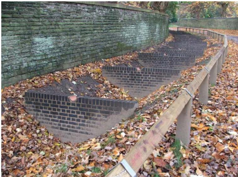
**FIGURE 7. COMPLETED STEPPED TRENCH SYSTEM ON MAYFIELD ROAD**
